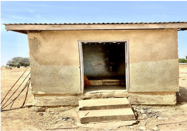
Figure 3 A toilet facility in a school. Source: (Fieldwork, 2022).
