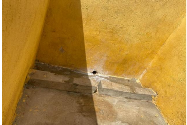
Figure 6 A urinal pit
