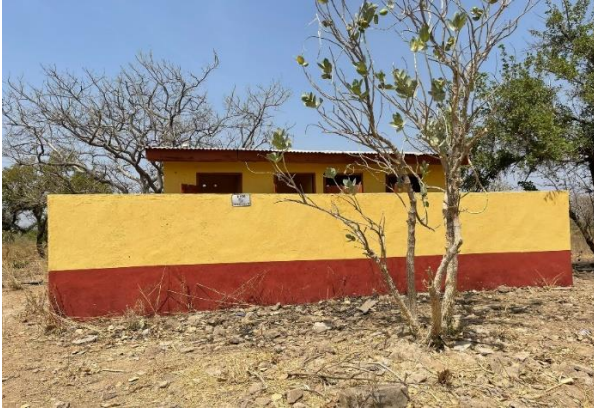
Figure 5 Newly constructed facility for both girls and boys, with functional doors.
