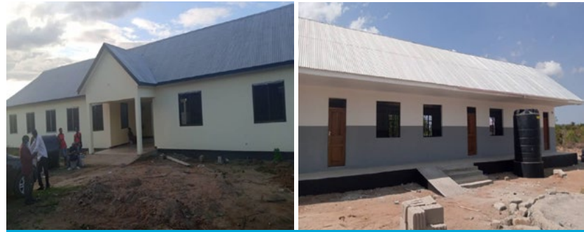
Boko Timiza dispensary building and Classrooms block at Viziwaziwa Secondary School
