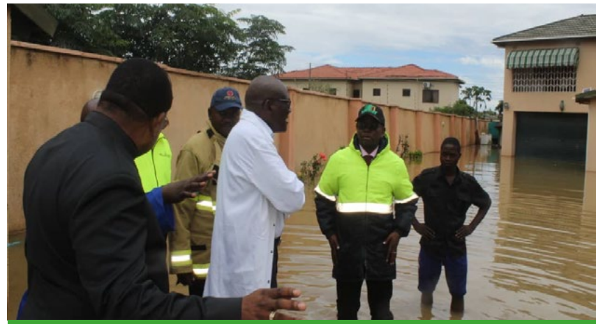
Flooding in Parts of the Lusaka City as a result of poor drainage system and poor Waste management
