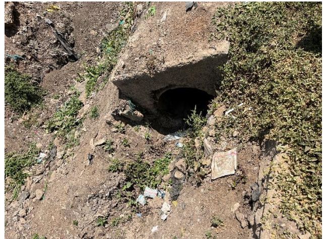
Figure 7 Narrow drainage culverts.
